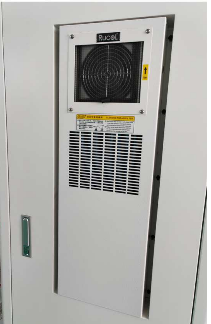
Heat exchange to keep cabinet clean and reliability
